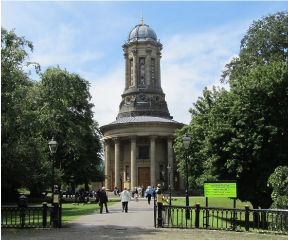
Grade 1 listed Saltaire URC, built in 1859 from local stone with an ashlar finish. The main part of the church is roofed with Welsh slate and has large plain windows.
