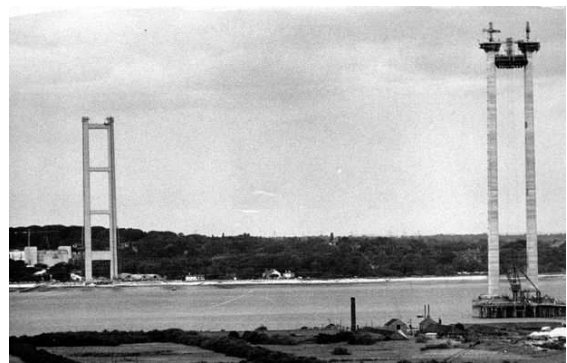
Humber Bridge under construction
