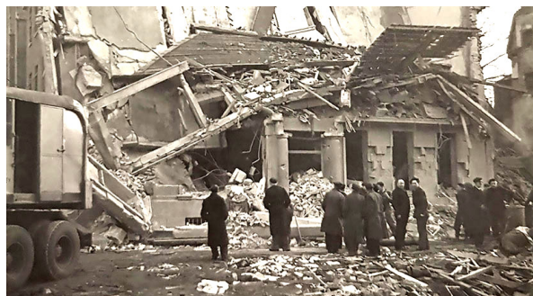
People gather to inspect the damage
