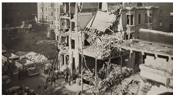
Damage to Presbyterian Church House
