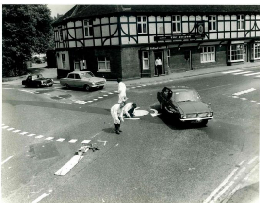
The Benfleet mini-roundabout being installed in May 1970
