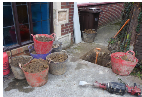
One of the holes for the branch to the vestry toilet
